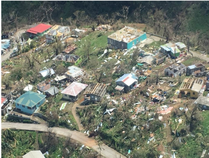
Damage from Hurricane Maria, Dominica, 2017.
