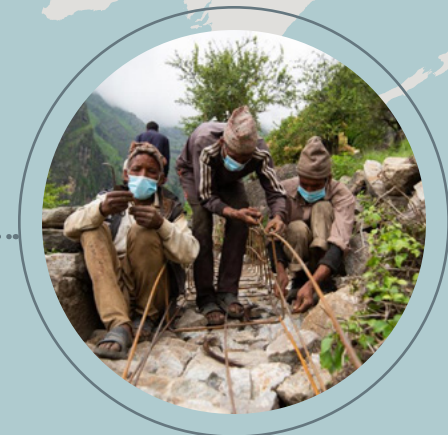
NEPAL: Community members rehabilitate a water canal in Situ Matela, a remote village in Nepal's Kalikot District. With BHA support, Mercy Corps provided materials, training, and technical advice to facilitate the rehabilitation project, which will ensure access to water for planting even during the region's dry seasons. Photo courtesy of Mercy Corps
