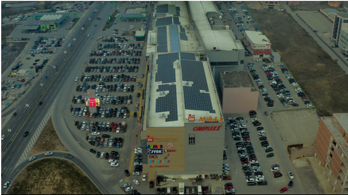
Figure 12 Albi Mall 500 kW behind the meter solar PV installation
