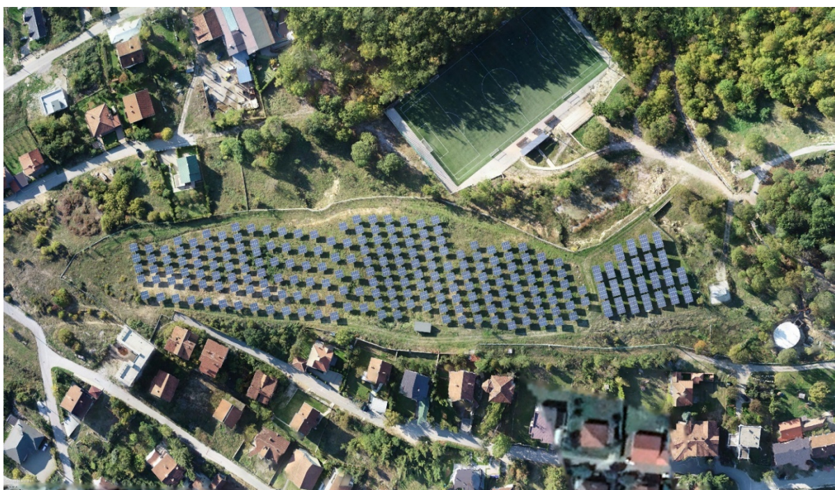
Figure 18 ONIX Spa, Banja e Pejës, Istog, 500 kW Solar PV based on Feed-in Tariffs
